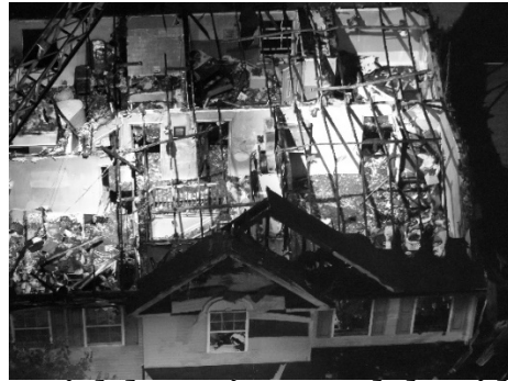
Aerial drone image, alpha side
