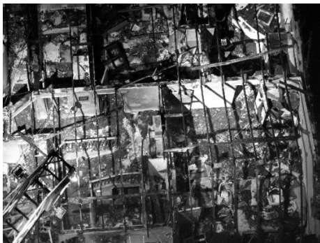
Aerial drone image, roof from alpha side
