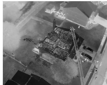
Aerial drone image, bravo side
