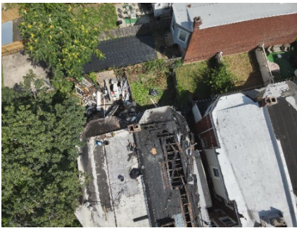
Photo 8. Aerial view of roof and side Charlie
