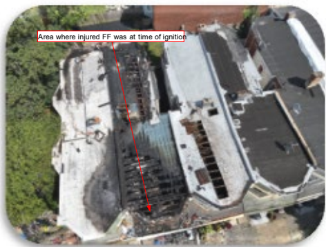
Photo 3 View from where the fire ignited from the cockloft. (FIRE Team Photograph)
