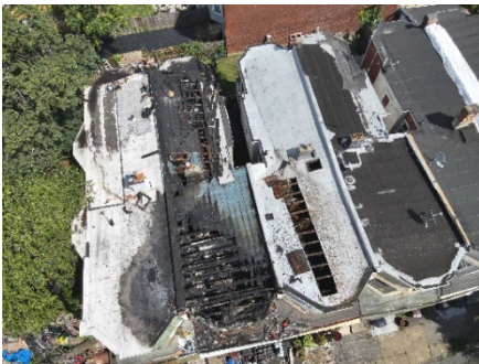
Photo 6. Aerial view of the roof from side Alpha
