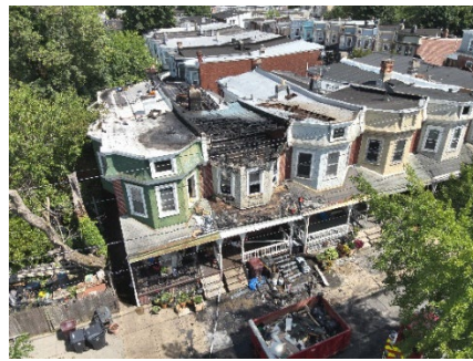
Photo 7. Aerial view of cockloft and roof
