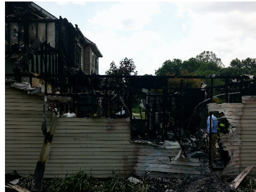
Photograph 4 Bravo Side View of Garage
